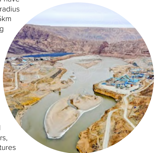
Yangqu dam under construction. Source: Radio Free Asia, 12 April 2024, via citizen journalist.
